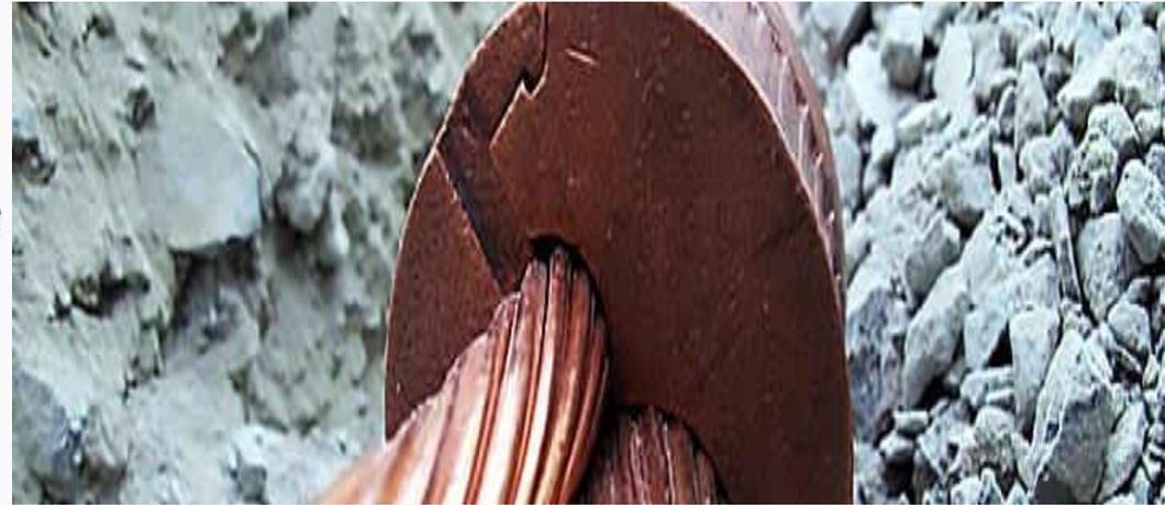
**Dissipation resistance  $R_A$**  of an earth electrode is the resistance of the earth between the earth electrode and the reference earth.  $R_A$  is in practice a real resistance.
